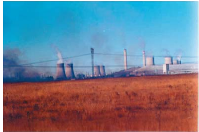
A smoky view of Sasol's Secunda plant
